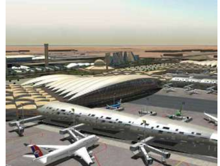
Riyadh Airport, K.S.A
